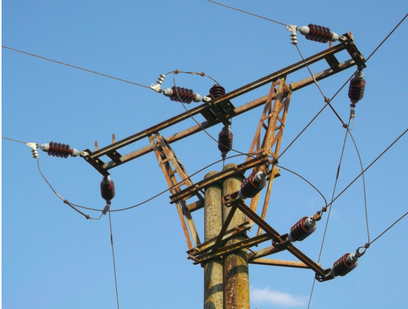
Figure B.1: Branch pole of 22 kV line with many exposed jumper wires used in Slovakia.
