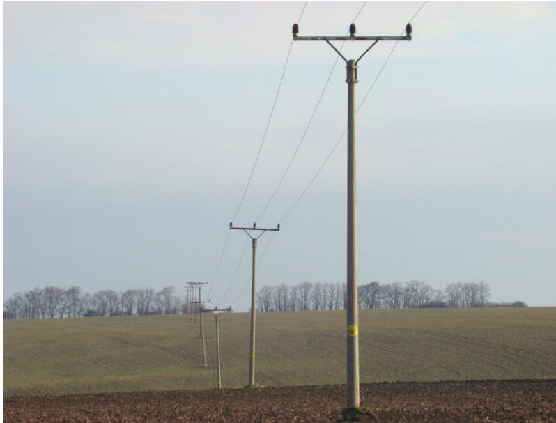
Figure A.3: Medium voltage pole of 22 kV distribution line in Slovakia. Source: Raptor Protection of Slovakia
