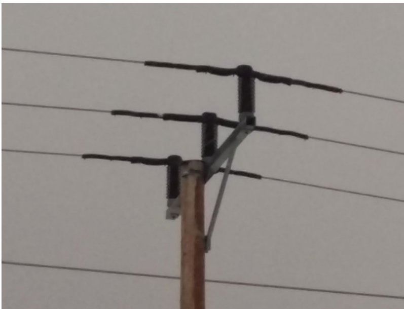
Figure C.2: Insulation caps for pin-type pylons in Sweden. Source: BirdLife Sweden
