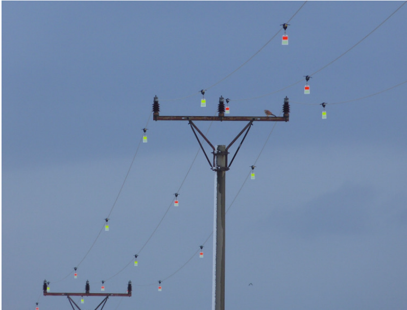
Figure D.3: FireFly Bird Diverters include an orange and a yellow part that reflect sunlight during the daylight hours and alert approaching birds to an obstruction in their flight path.
