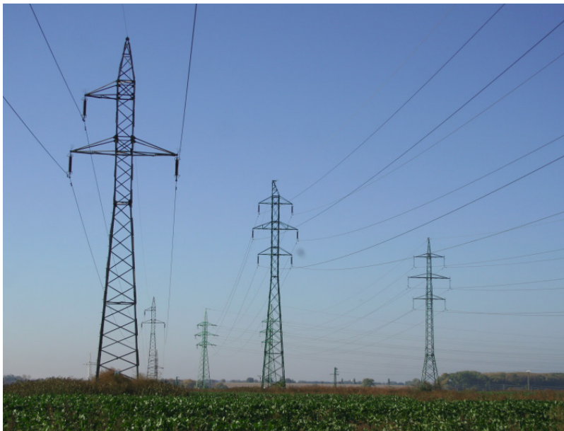
Figure A.2: High voltage pylons of 110 kV distribution line in Slovakia. Source: Raptor Protection of Slovakia
