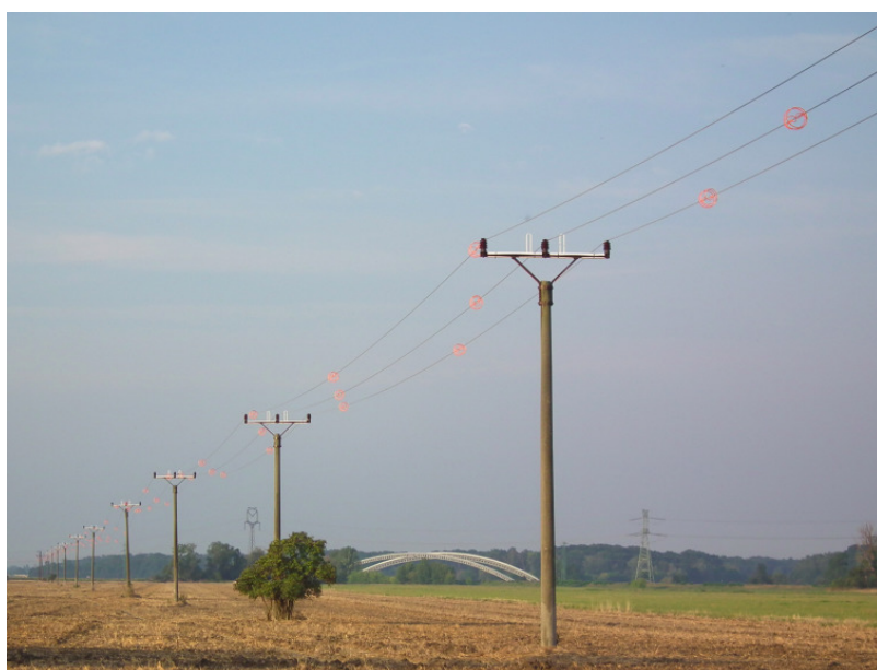
Figure D.2: Fully protected medium voltage line in Slovakia. Orange spiral diverters increase the visibility for bird species in their feeding area. Source: Raptor Protection of Slovakia
