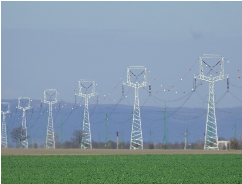
Figure D.6: Avian marker balls provide visual warning for planes but are also effective for bird protection. Source: Raptor Protection of Slovakia
