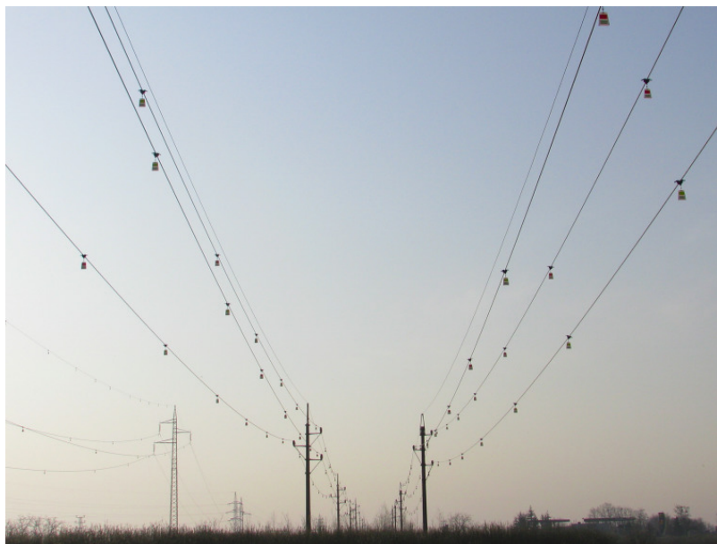
Figure D.1: Dangerous sections of 22 kV lines marked with FireFly Bird Diverters. Source: Raptor Protection of Slovakia
